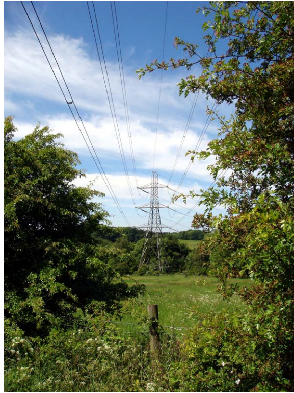
Photo 1 - Sample Caption - Power lines near sample customer
